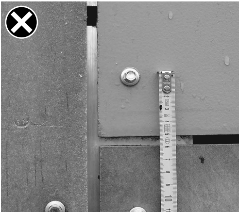
Faulty Roster Dilation
