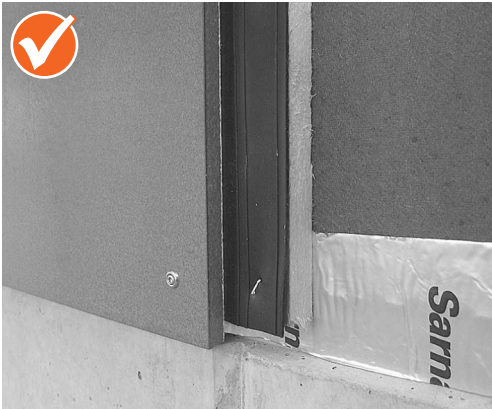
Correct use of the rubber tape
