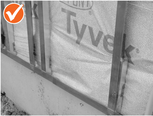
Correct way of mounting the L-profiles along the vertical gap
