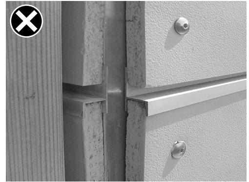
Base under the Boards not leveled
